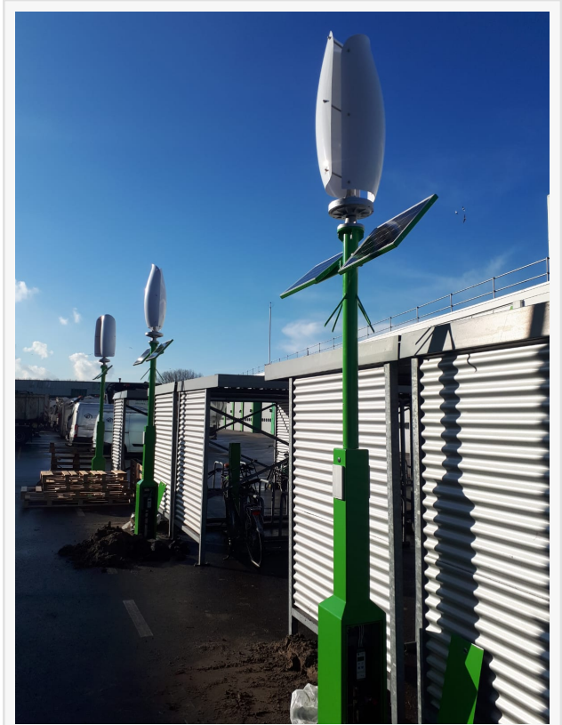
Wind and Solar E-bike Charging Poles
