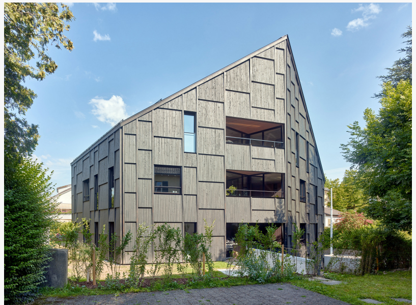
Gardenfacade of L329 Zurich, Switzerland - Photo by Juerg Zimmermann, Zurich
