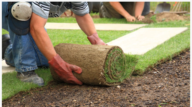
Primrose Landscaping and Snow Removal Ltd. Prepared For The Spring Season
