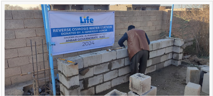
LIFE team member laying bricks in the construction of the water station.
