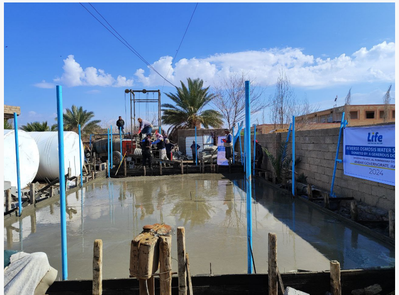
The construction of the water station.
