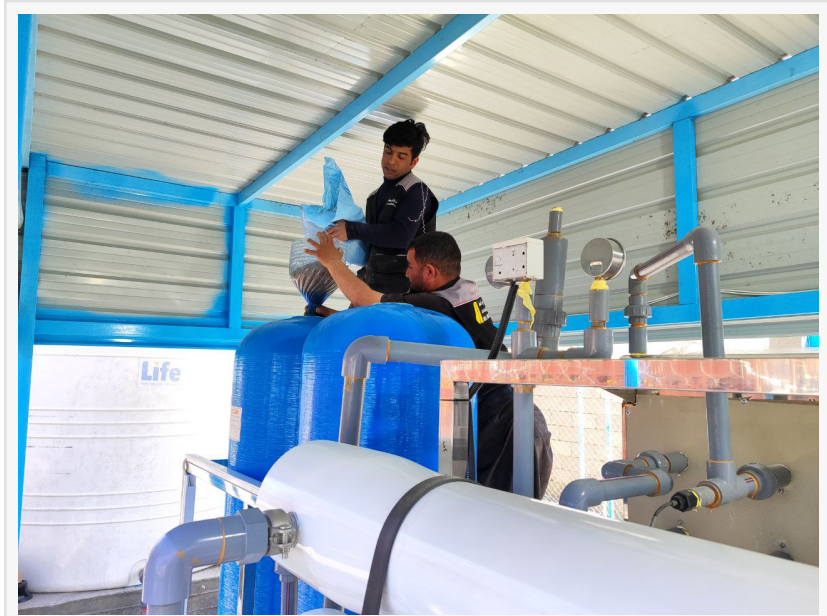
LIFE Team member putting the final touches on the water station.
