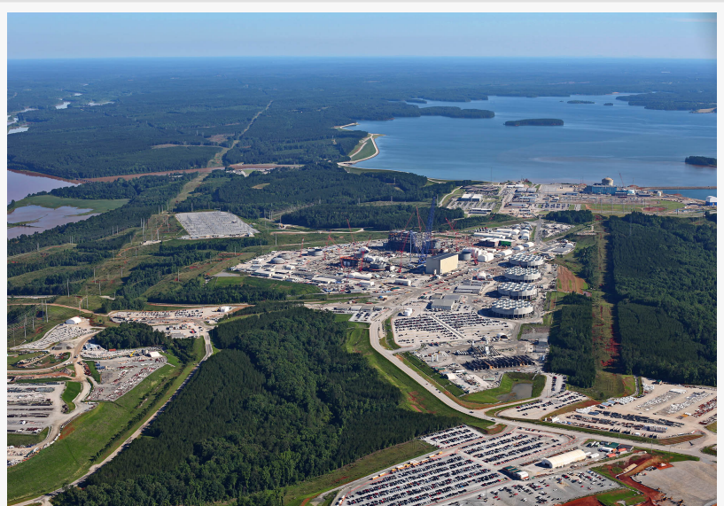
Aerial shot of Dominion Energy's V.C. Summer site north of Columbia, SC, with two terminated Westinghouse AP1000 reactors in foreground and single operating unit in background. Photo ©High Flyer 2017
