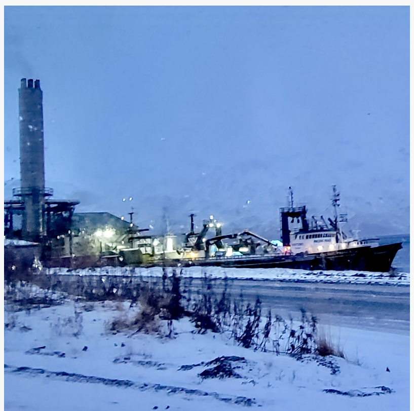
Westward Dutch Harbor Seafood Processing Plant
