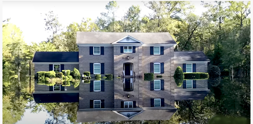
The Ridge family has restored the property after a massive flood several years back.
