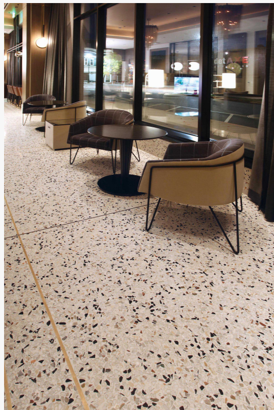
MARBLE aggregates in larger-than-standard sizes distinguishes the traditional Venetian-style terrazzo.
