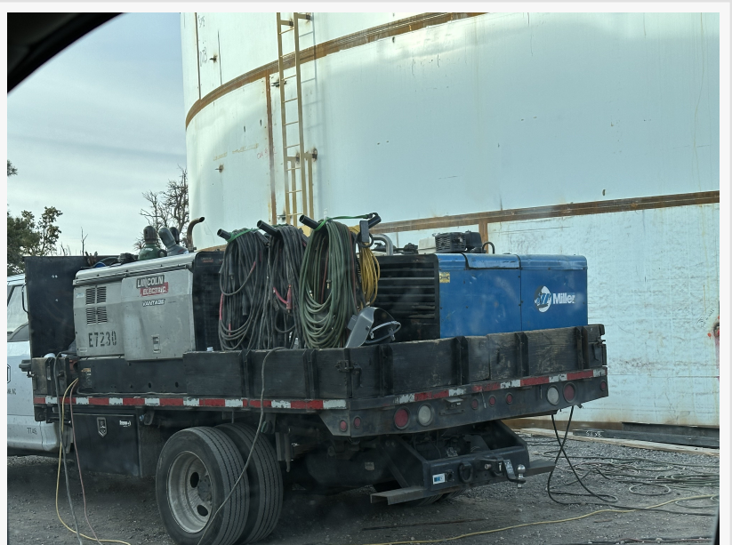
Expert AWS CWI Inspector from AWSCWI.COM Conducting Precision Tank Welding Inspection
