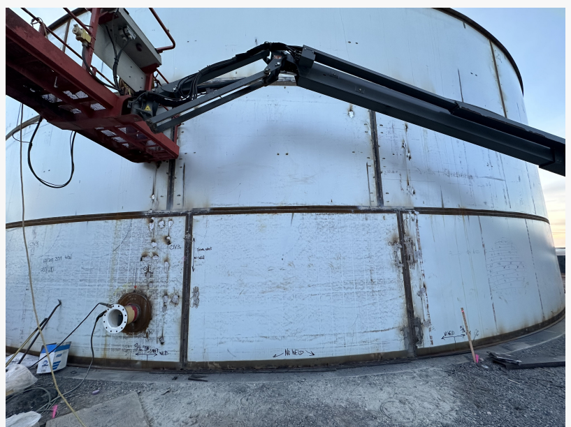
AWSCWI.COM's Certified Inspector in Action: Ensuring Tank Welding Integrity Nationwide
