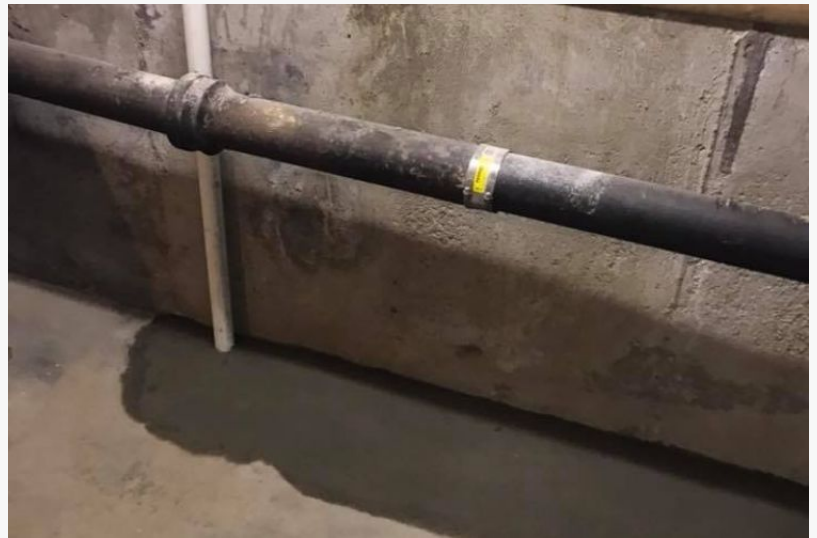
before waterproofing services in Rhode Island home
