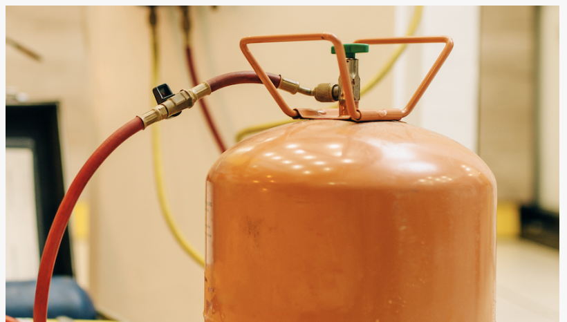
Propane tank in a kitchen.
