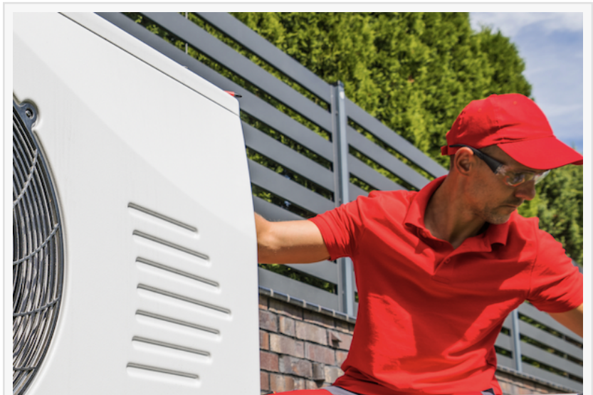
Man installing heat pumps.
