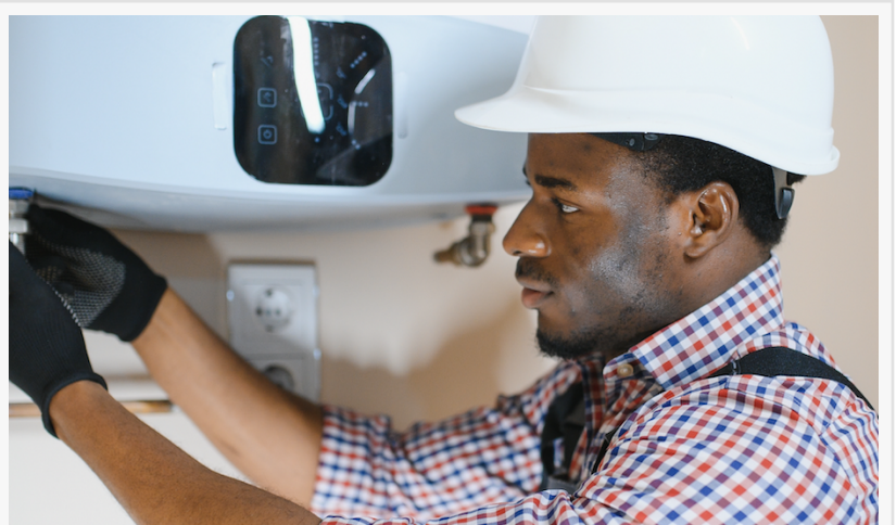
Man fixing a boiler.
