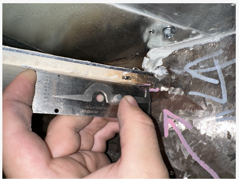
Inspecting for weld undercut with precision at AWSCWI.COM.
