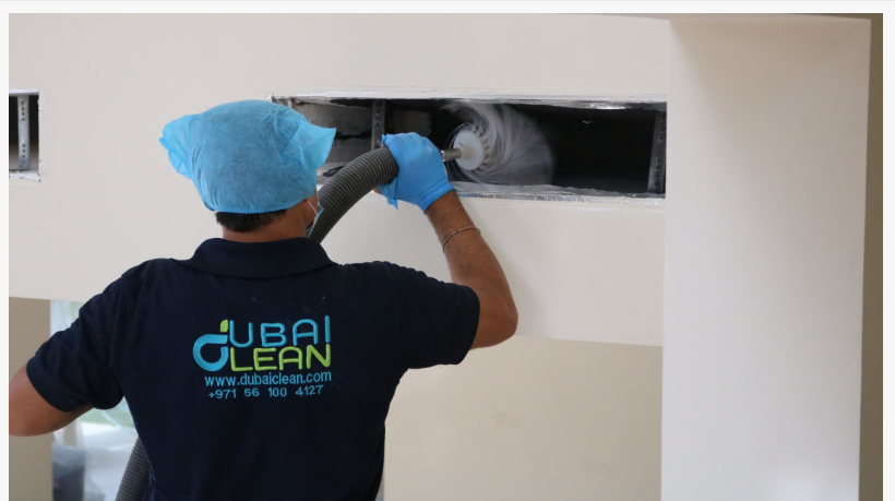
DCS DubaiClean AC Duct Deep Cleaning Services Dubai
