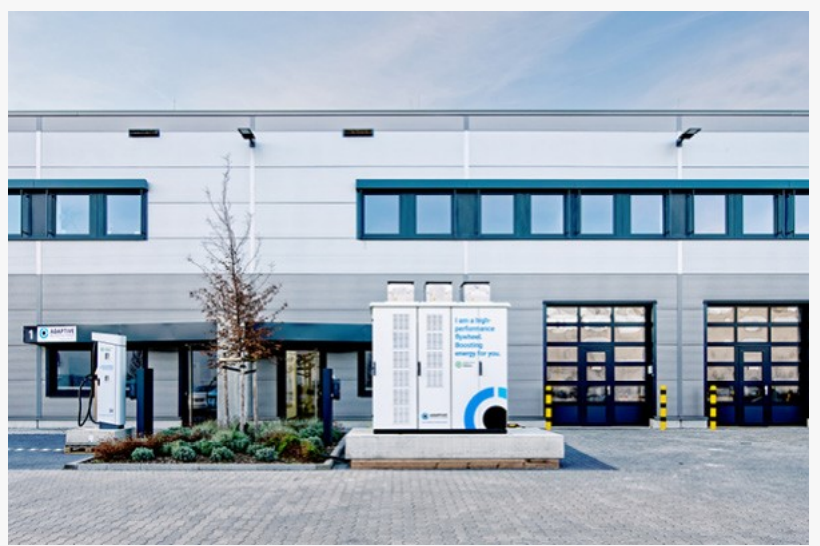
Adaptive Balancing Power Headquarter in Pfungstadt Germany c ABP
