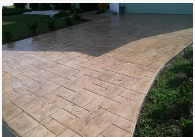
Beautiful custom concrete work
