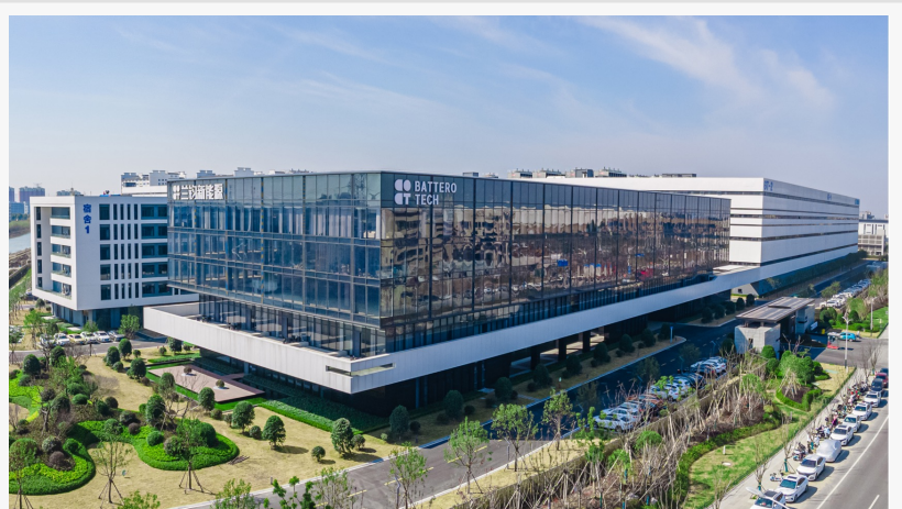
BatteroTech Headquarters Jiaxing
