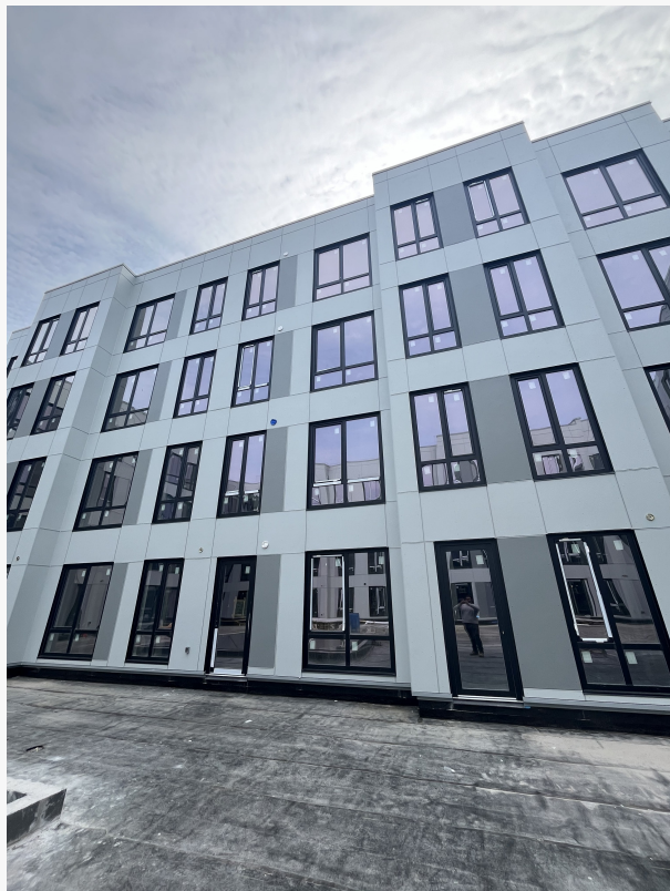
Exterior work on The Forte's facade along Anderson Street. Hackensack, NJ.
