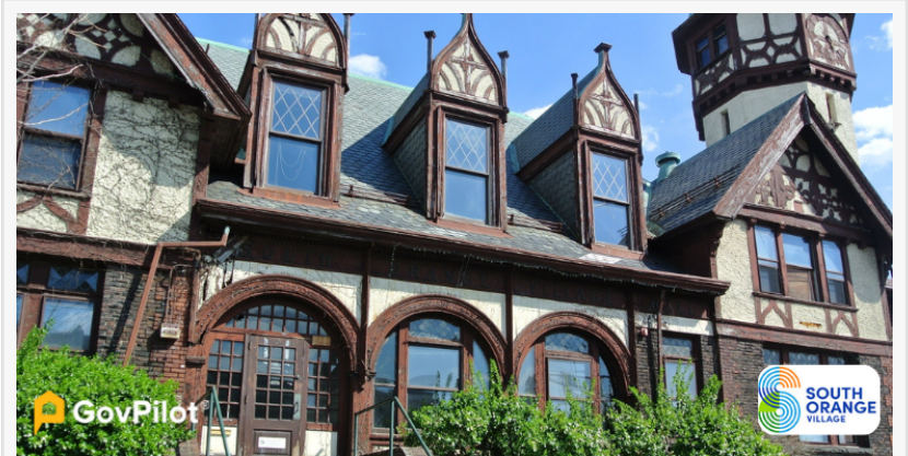
South Orange, NJ Deployed Life Hazard Module With GovPilot
