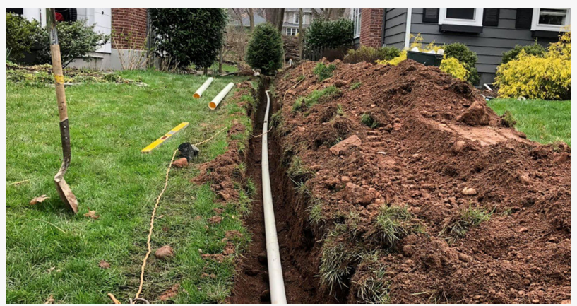
Yard Drainage Installation
