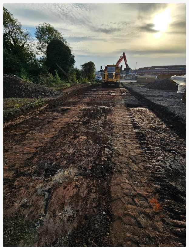
Works underway on Terra Firma Energy's new BESS Project
