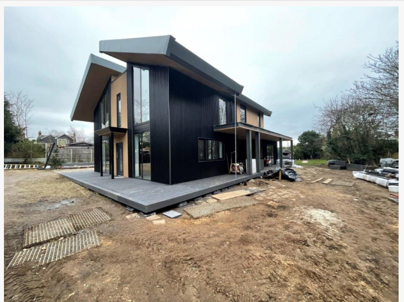
SIPS house extension
