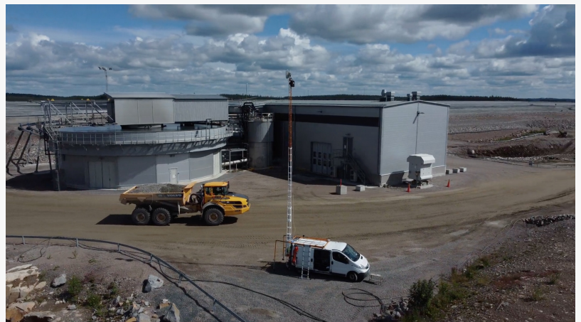
5G network deployment in action at Garpenberg Mine
