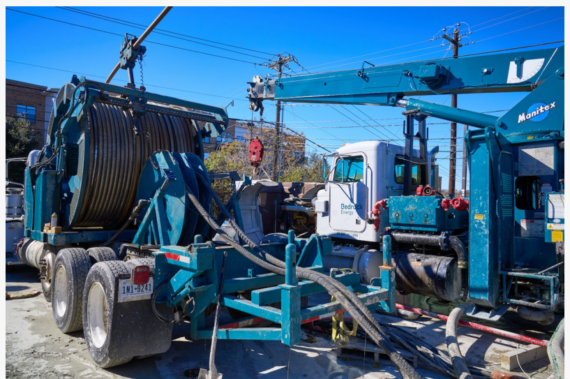
Drilling rig at Penn Field
