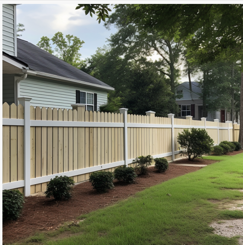
A Privacy Fence installed by SecureEdge Fence Installation in Augusta, GA
