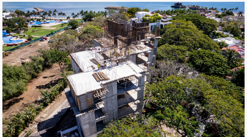
Kovay Gardens Marine Diamond New Construction
