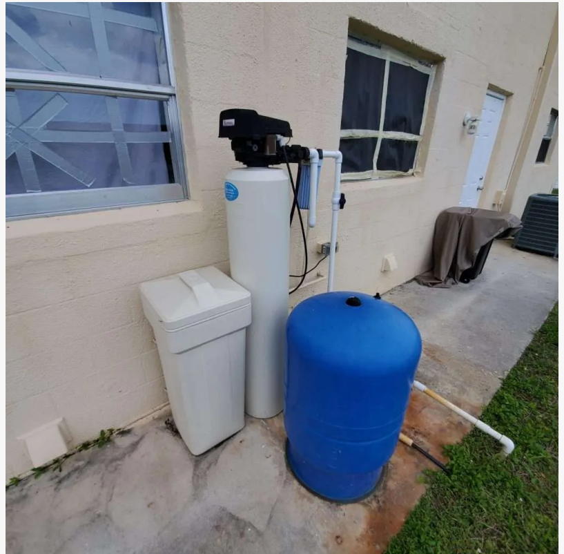
Installs home water softener
