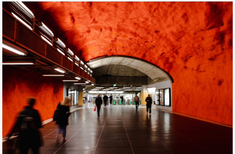
Solna subway station, Stockholm
