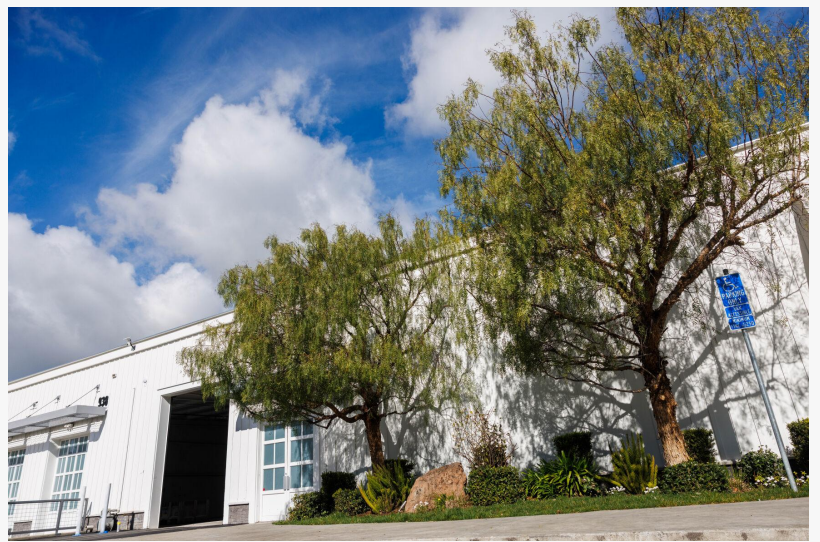
The new facility, located at 938 Kaiser Road in Napa, expands the Food Bank's capacity to 18,000 sq/ft
