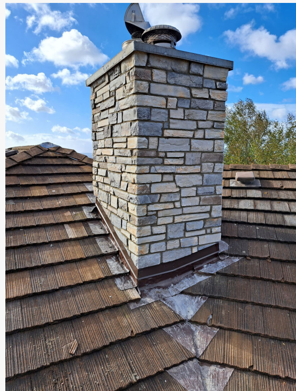
Stone and Brick Chimney Cap Installations
