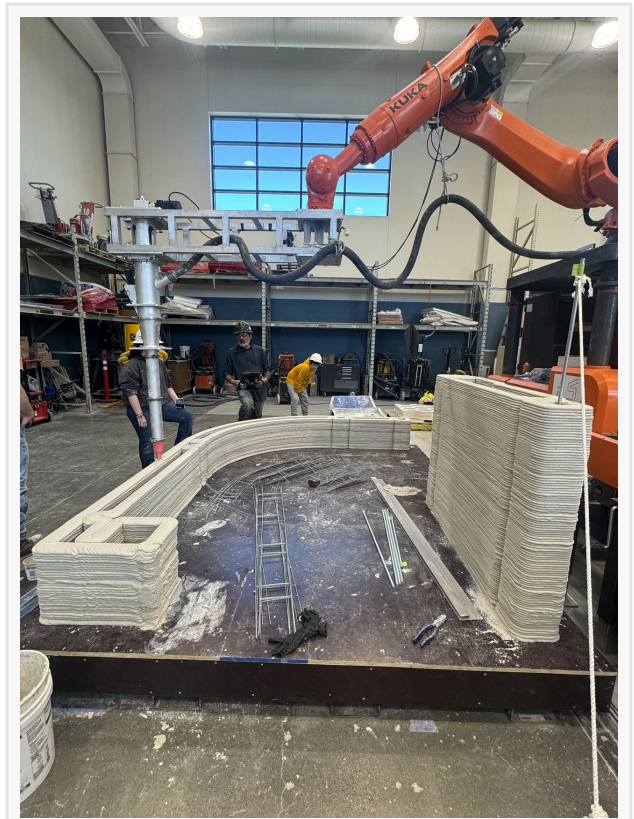
RIC-M1 Pro 3D concrete printing
