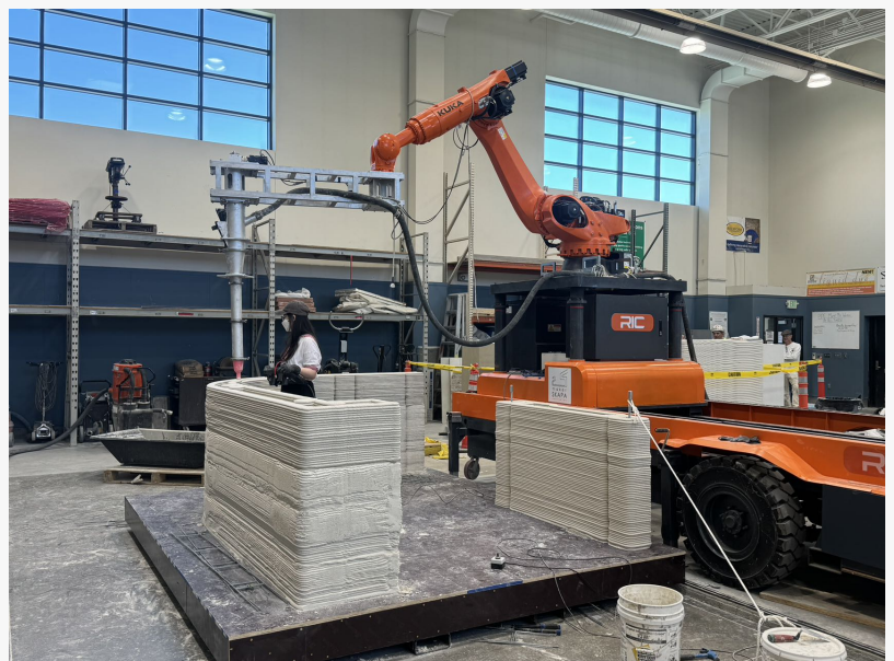
RIC-M1 Pro 3D concrete printing
