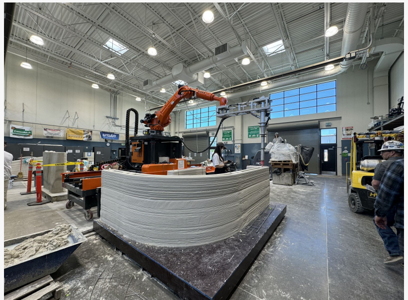
RIC-M1 Pro 3D concrete printing
