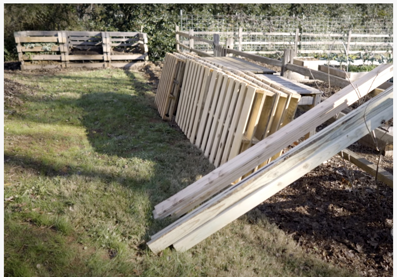
The project starts with nine recycled wood pallets, along with a variety of 1x6-inch and 2x4-inch boards.
