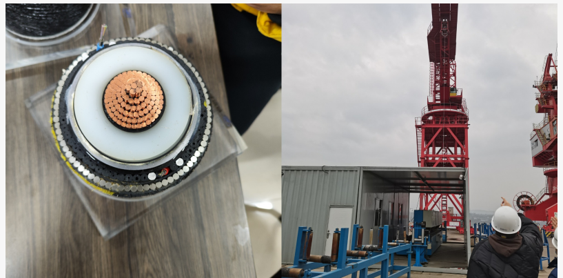
ZMS and TCN cooperate on the site construction of the submarine cable project and are accepting the quality of the submarine cable.
