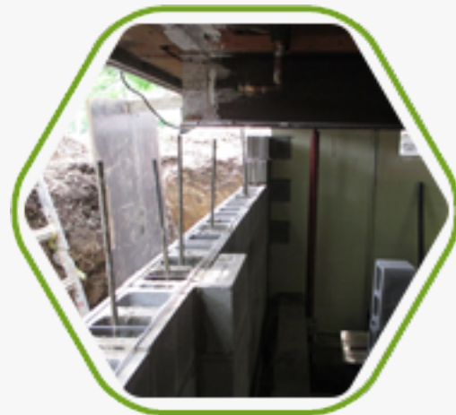
Basement Waterproofing Service
