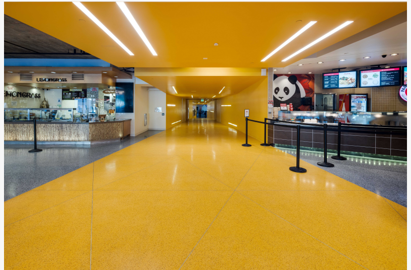
TERRAZZO flooring was used to create a yellow tunnel at the renovated Price Center. Photos: Nathan Padilla Bowen
