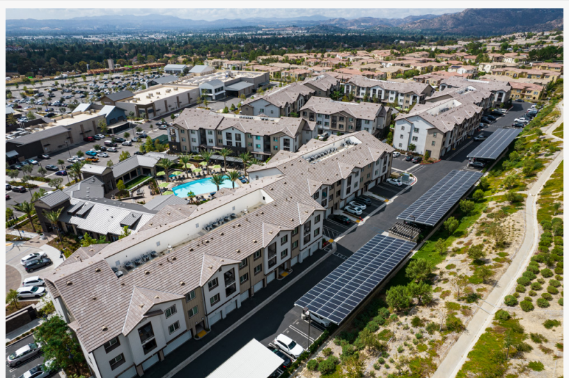
Carports with solar panels produce energy for a community in Porter Ranch, California
