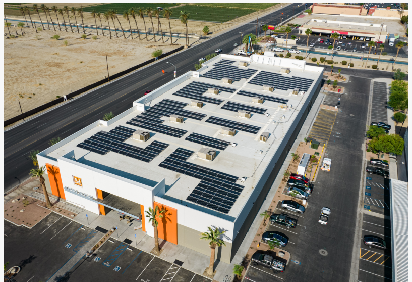
Solar keeps a furniture showroom bright and cool in Indio, California.
