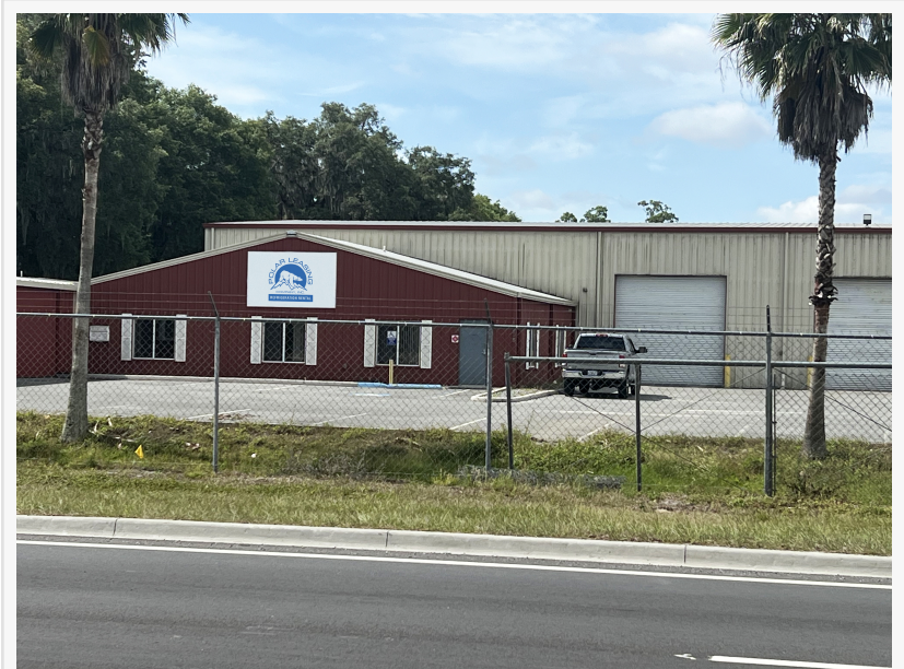
Polar Leasing is growing operations with a new facility in Sumterville, Florida. This marks the company's initial real estate venture beyond its Fort Wayne, Indiana, headquarters.
