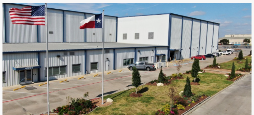
National Strand's new, state-of-the-art 55-acre facility in Baytown, TX
