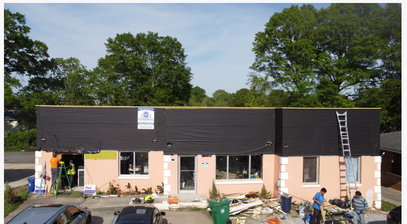
Constructing A Commercial Property in Atlanta Georgia
