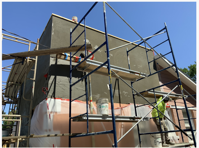
Renovating a Commercial Property
