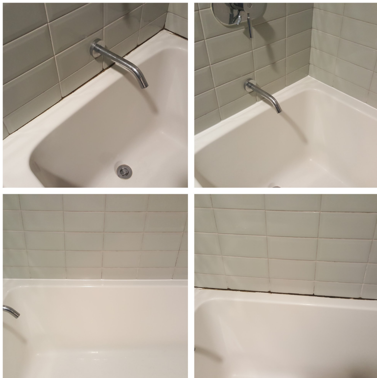
Before and After bathroom shower/tub grouting repair
