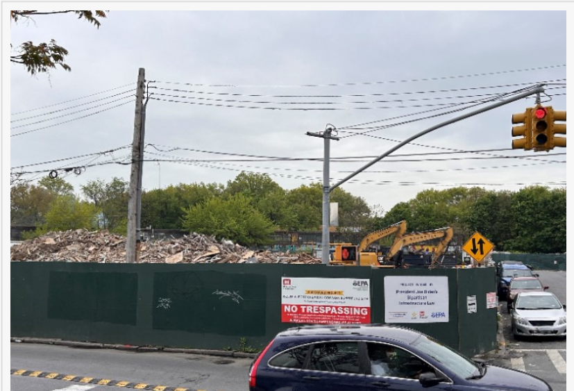
Demolition Currently Underway
