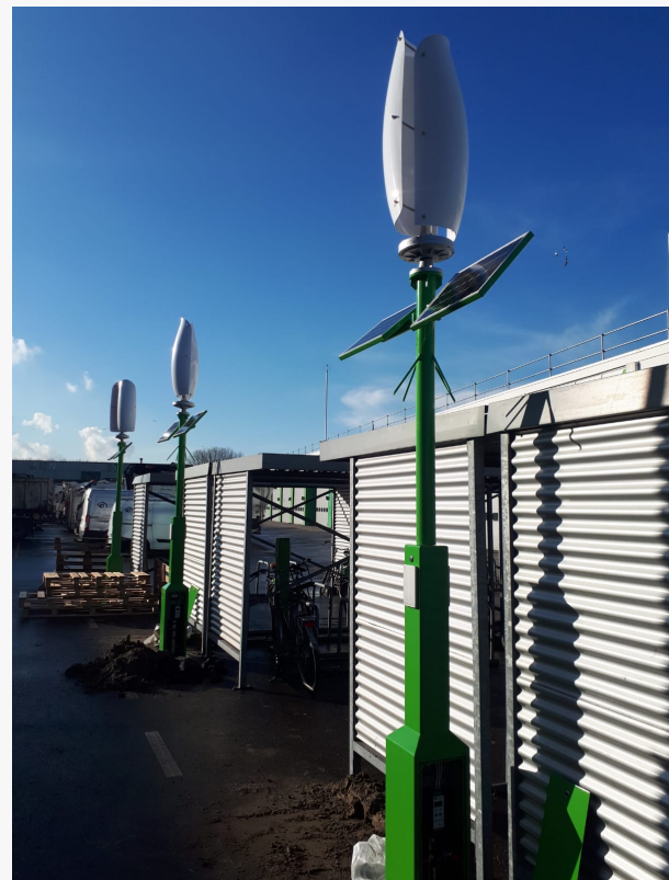
Wind and Solar E-bike Charging Poles
