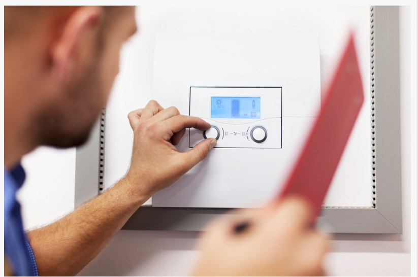
Tankless Water Heater Installation in Tucson
