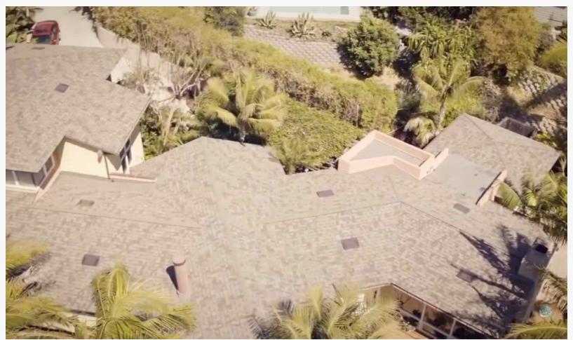
RC Solar & Roofing - Re-roof
