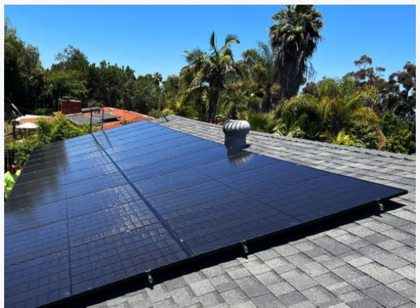
RC Solar - Panels Installed
