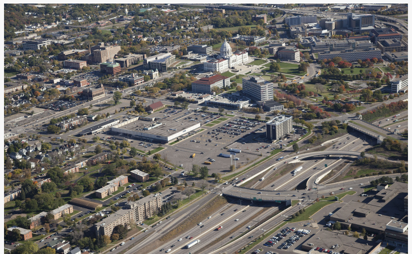
A bird's-eye view captures the Sears building, parking lot, and surrounding area
