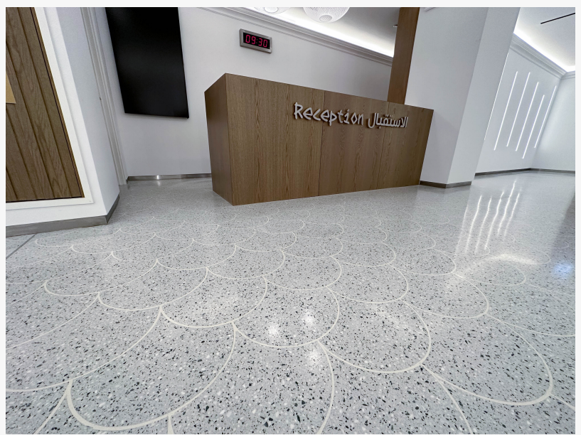
TERRAZZO designed with an innovative pattern of arches distinguishes the winning installation. Photos: Louis Thomas
