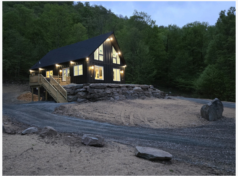
New Construction Chalet in Sullivan County NY
