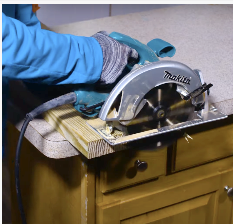
A circular saw is used to cut the boards to length.
