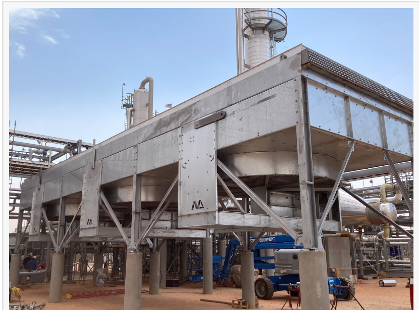
Installed air cooled heat exchanger, engineered and built by North American Air Exchanger
